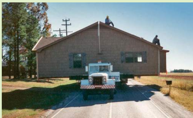
Hollis Kennedy House Movers
